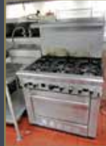
(18) US RANGE 6-BURNER RANGES W/CONVECTION OVEN
